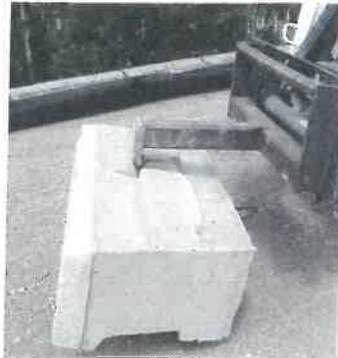
A block being set in place with a skid steer.
